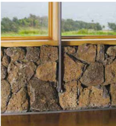
Steel supports (left) tie the structure down to the lava-rock base. Custom details include rolling doors (below left) that open the walls to wide Pacific views, as in the kitchen/dining area (above).
