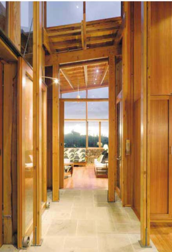
Metal cross bracing, as in the kitchen (above) and corridors (left), helps stabilize the roof structure for high winds and seismic events. Eucalyptus paneling and cabinetry, along with stone floors, add warmth to 16-to-18-foot-high passageways (left).
